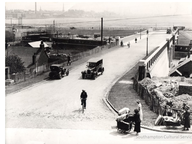
View from what is today Central Station Bridge towards the construction work, about 1930.
